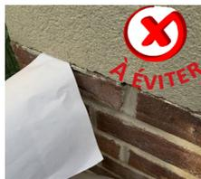
En façade, joint manquant (source qualiconstruction.com)
